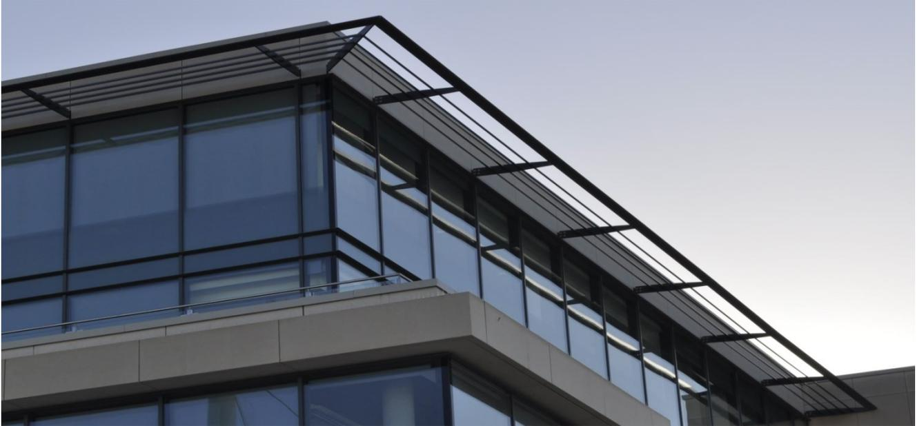
**Emtec extruded aluminium fins are used for solar shading of glazed facades. Benefits can include a reduced heat load on the building leading to increased occupant comfort, optimised natural light and a reduction in the whole energy consumption of the building.**
