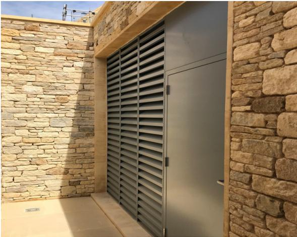
EMTEC LAAC 15-105 Acoustic Louvres can be installed as individual units or by bolting more than one unit together (horizontally or vertically) openings of any size can be accommodated. Each louvre has a robust outer framework which acts as vertical mullions and horizontal transoms when several units are fixed together. If a continuous blade effect is preferred this can also be supplied.
