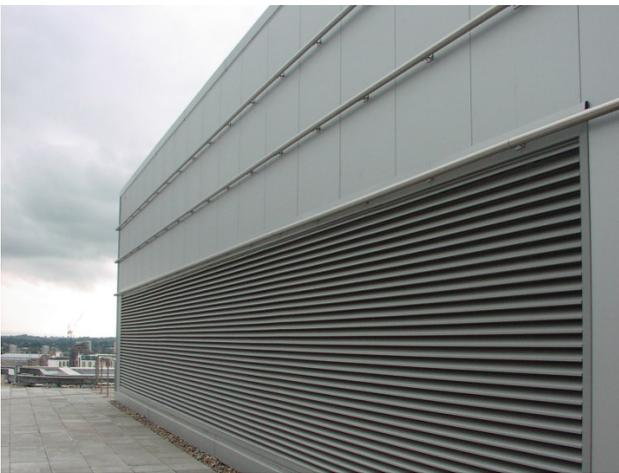
minimises the resistance to airflow whilst the incorporation of water traps ensures that the ingress of rain is reduced.
